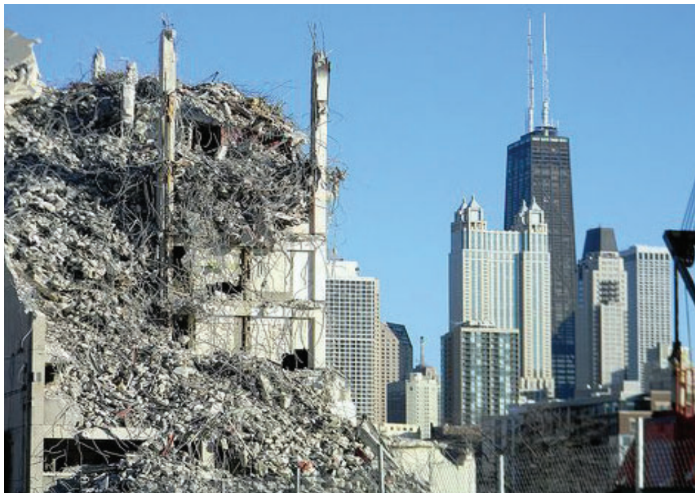
Fig (19): The Cabrini-Green Project Demolition
