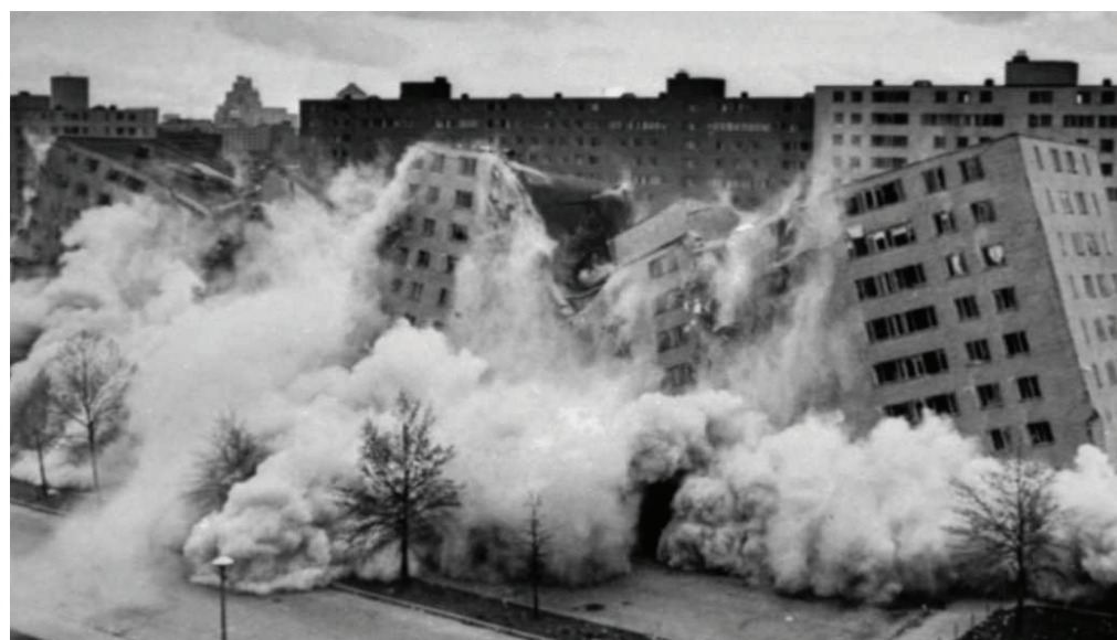
Fig (17): Pruitt Igoe Public Housing Demolition
