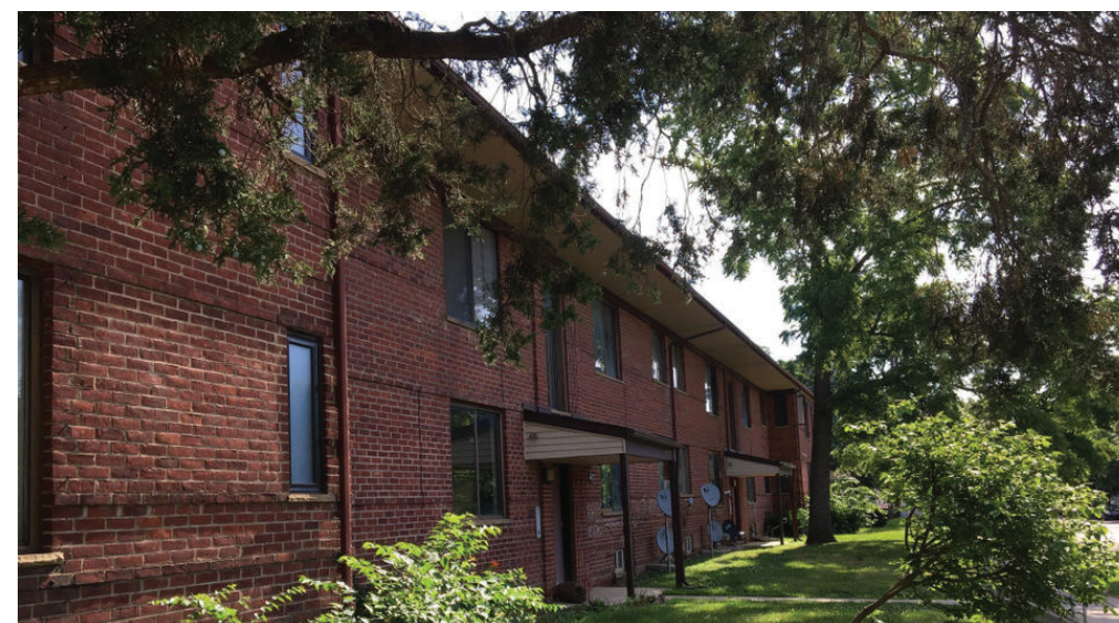
Fig (21): Building at 701 Henry St., Ann Arbor
