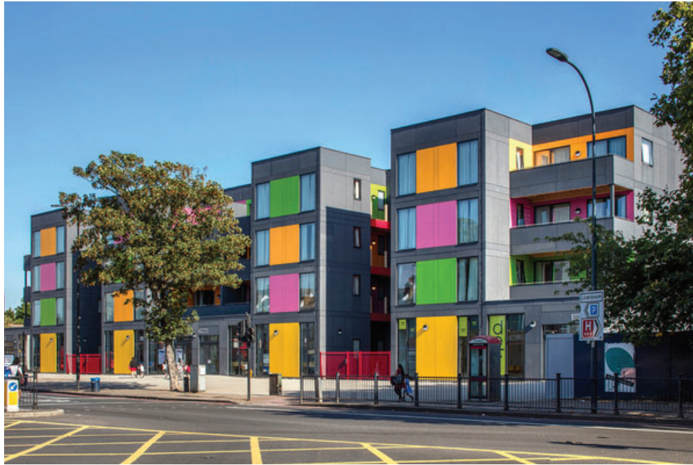
Fig (34):Ladywell Centre Volumetric Development
