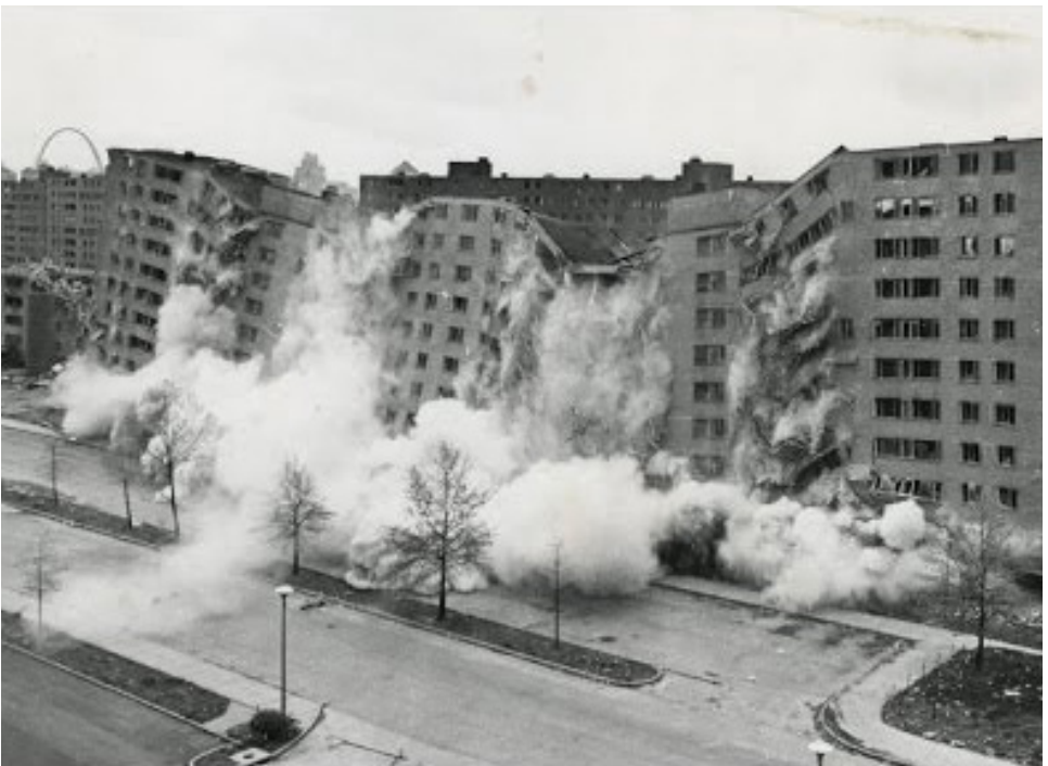
Figure 4, Demolition of Pruitt Igoe
