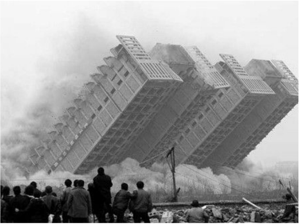
Figure 3, Demolition of Pruitt Igoe
