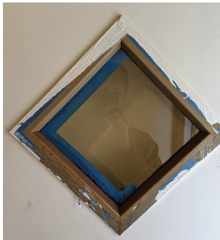
Figure 6.19 Closeup door paint peeling
