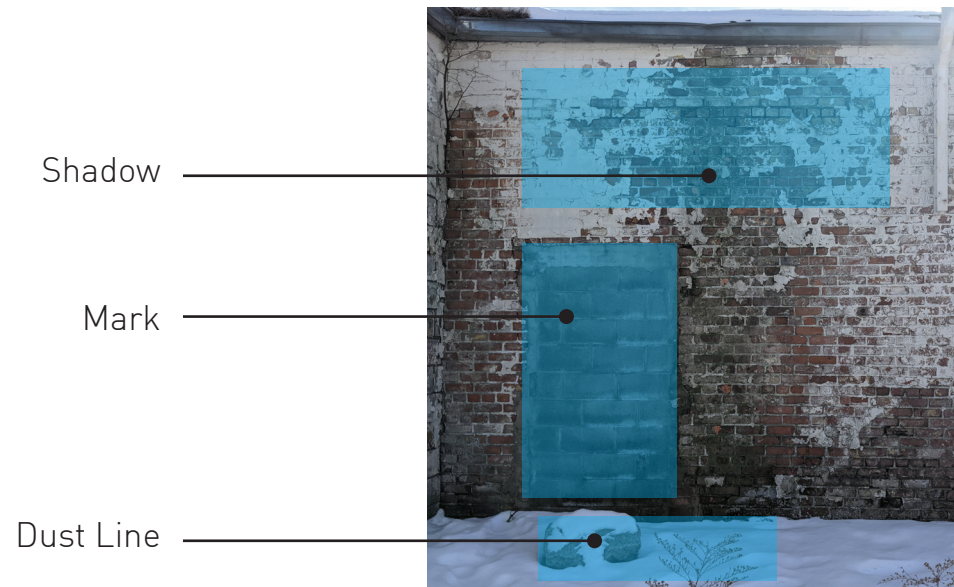
Figure 8.14 Image depicting Mark, Dust Lines, and Shadow on the building
