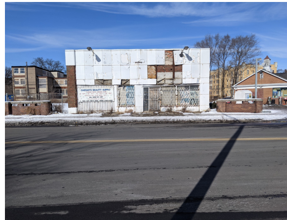
Figures 8.44-8.46 Images of building
