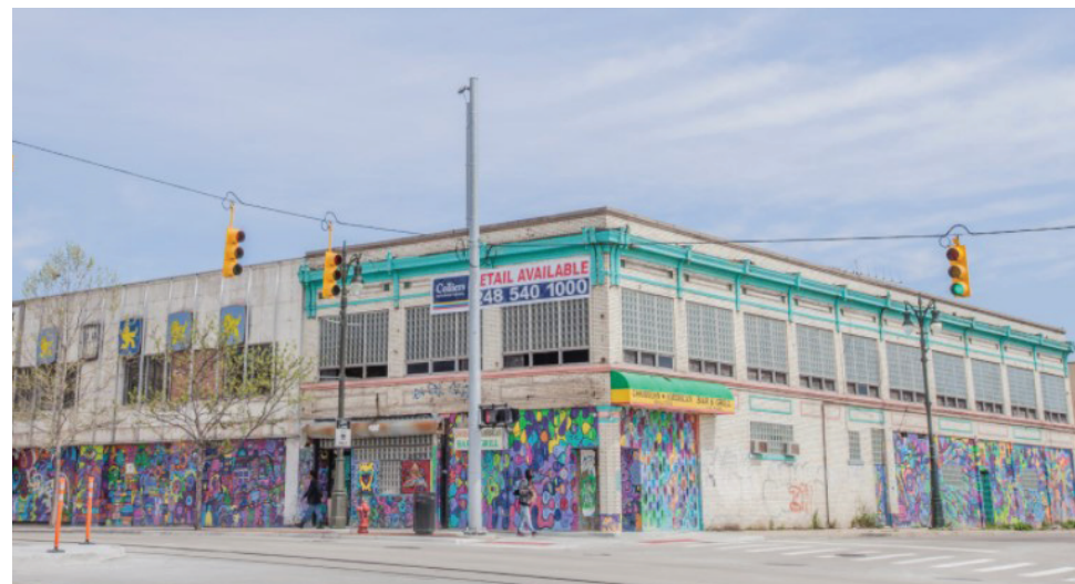
Figure 5.9 Old Baltimore Station building before its current use
