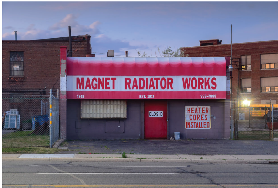
Figure 5.4 Old Magnet Radiator before being reused
