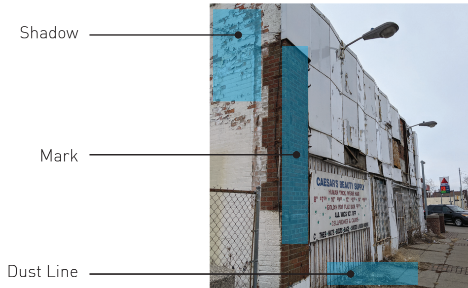
Figure 8.16 Image depicting Mark, Dust Lines, and Shadow on the building
