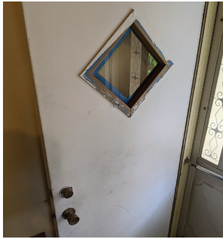
Figure 6.18 Side entrance door
