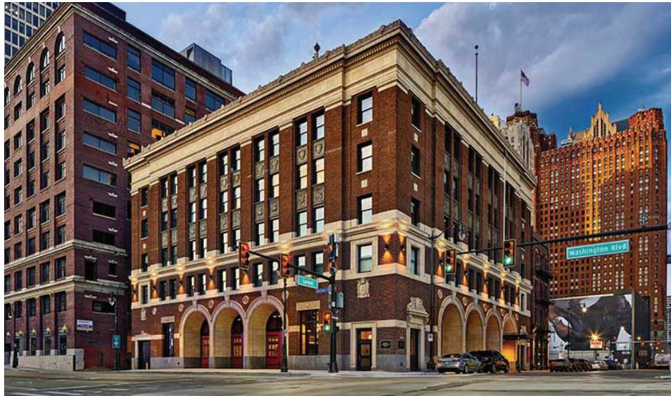
Figure 5.11 Current Foundation Hotel building after reuse implementation
