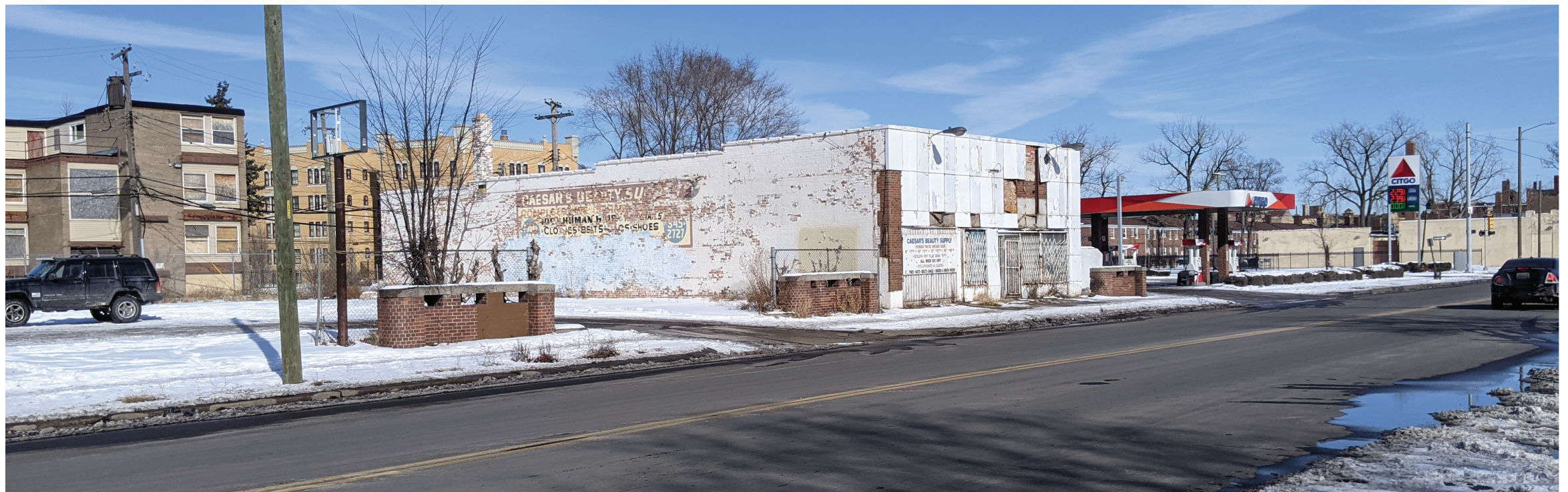
Figure 8.2 Image of 846 McNichols from the South West corner
