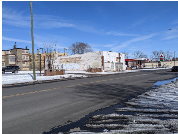
Figures 8.41-8.43 Images of building
