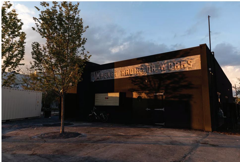
Figure 5.2 New Restaurant use located within old radiator shop
