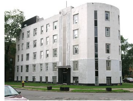
Figure 8.30 Image of apartment at Whitmore and Manderson
