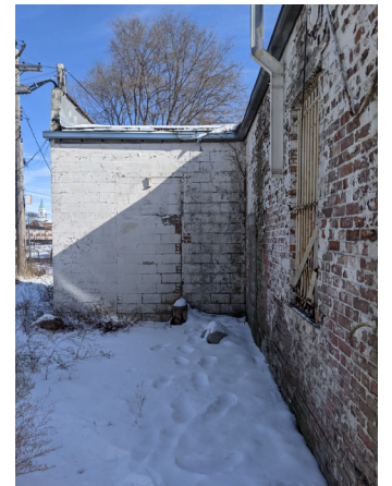
Figures 8.47-8.49 Images of building
