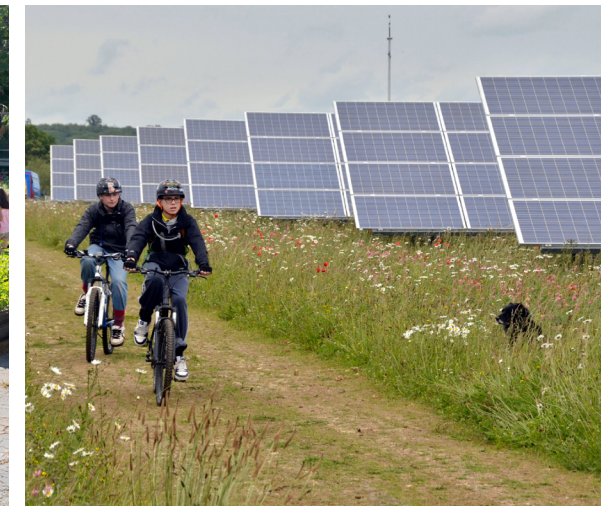
Community solar farm
