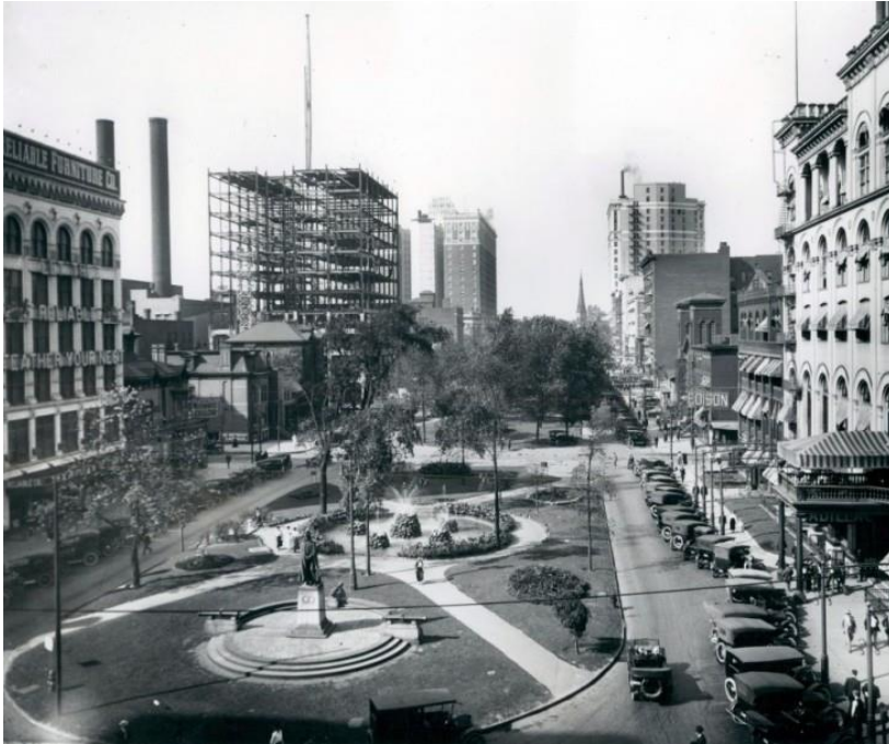
Figure 16: The construction of the Book Building which opened in 1917 (historicdetroit.org).
