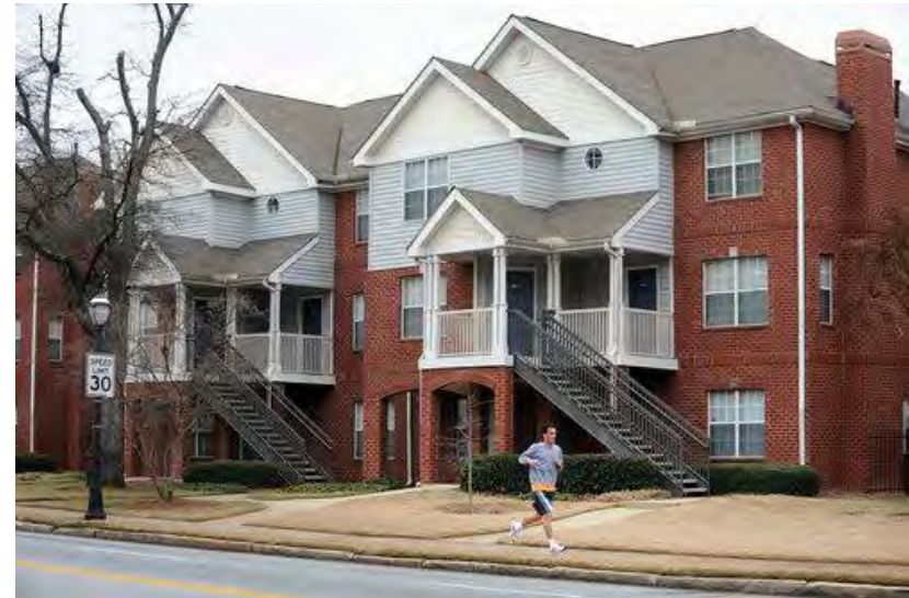
Figure 27: Centennial Place, Atlanta, Georgia Source: affordablehousinginstitute.org
