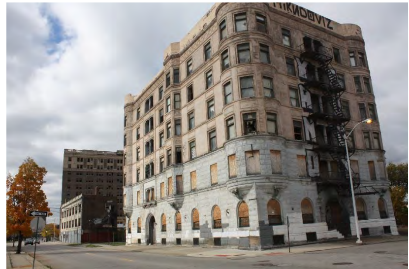
Figure 16: Vacant apartment building. (Temple and Park Ave.) Source: Authors
