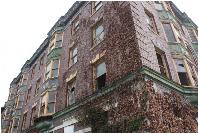
Figure 13: Vacant apartment building. (2nd Ave. and Charlotte St.) Source: Authors
