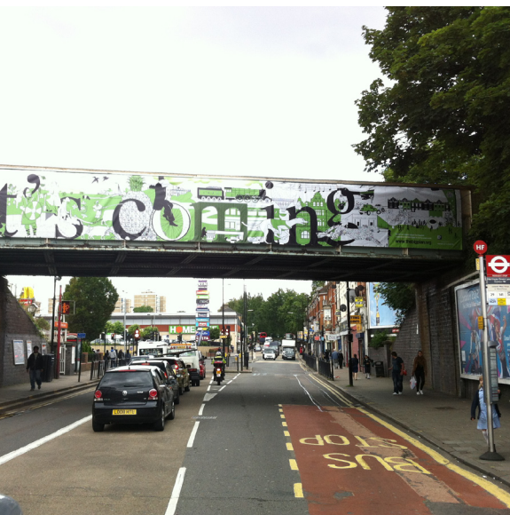
Fig. 206 Harringay Bridge in the London Borough of Haringey in north London, United Kingdom
