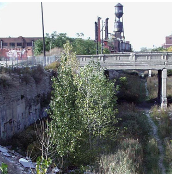
Fig. 46 Conditions of Dequindre Cut before greenway installation
