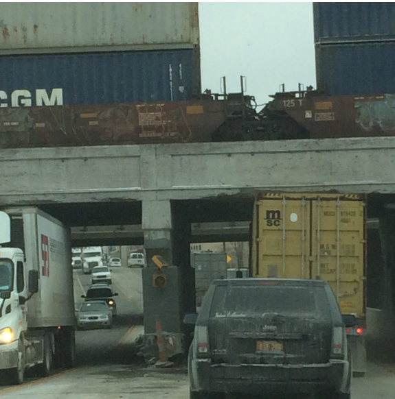
Fig. 64 Underpass along Vernor Highway for ICG and automobiles
