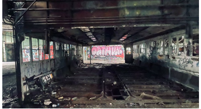
4 The echoing travels along the tunnel.
