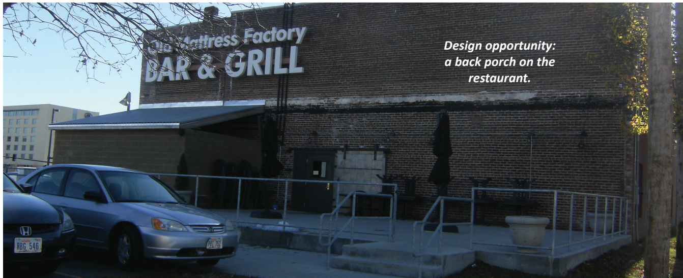
The East side facing the southern portion of the site.
