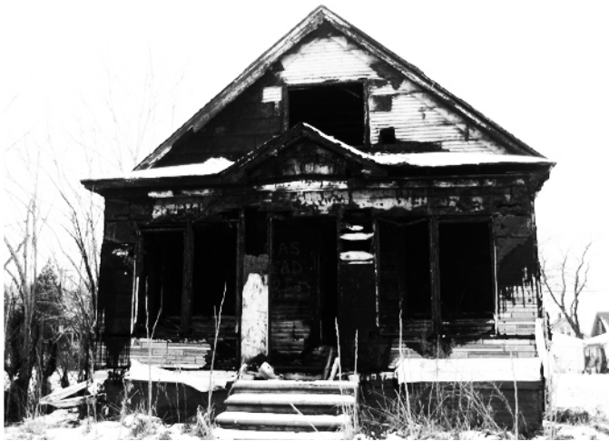
home in detroit, michigan destroyed by economical degeneration
