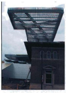
Market Street is a main East-West axis in the City of Akron the addition can be "sensed" by the traveler on this road even when it is directly blocked from view, this is done so by the grafted on cantilevered element Referred to as "the roof cloud" by the Architects. It Is constructed of a pronounced steel frame and steel grid panels that allow it to be semitransparent giving it a "light" demeanor, even though it is a very monumental structural element.
