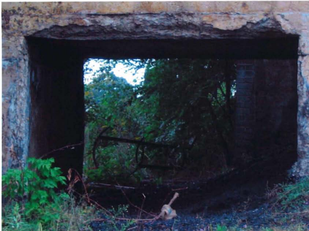
Figure 6.10 [above]– View of spalling concrete from the bridge’s structure Figure 6.11 [below] – view of brick peeling away to expose structural steel
