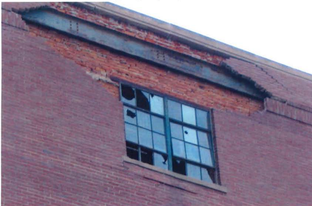
Figure 6.10 [above]– View of spalling concrete from the bridge’s structure Figure 6.11 [below] – view of brick peeling away to expose structural steel
