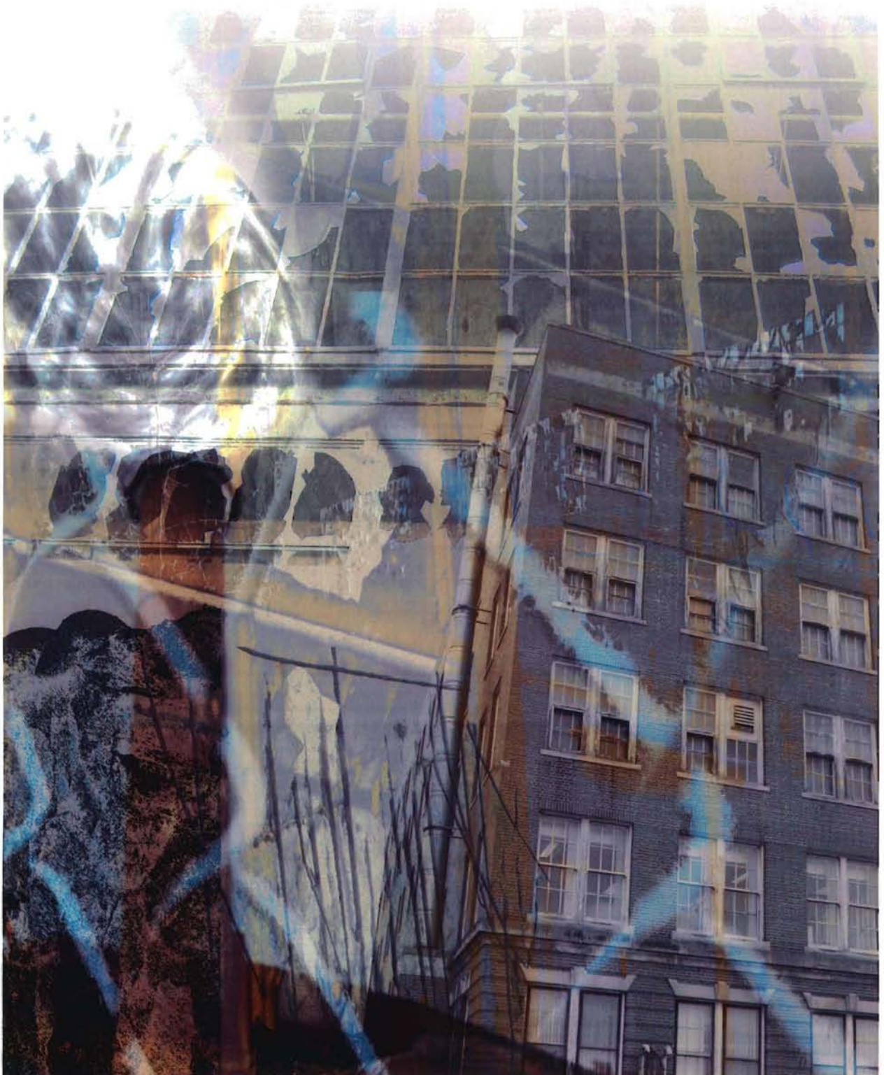
Figure 6.15 – Site photo montage
