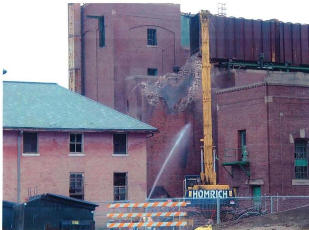
Figure 3.19 – The demolition of the power plant’s smokestack
