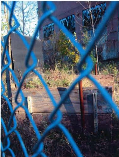
Figure 6.1 – View to powerhouse
