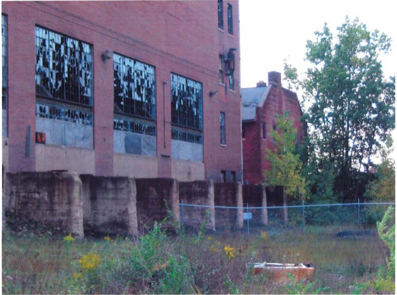
Figure 6.7 – View of the rear elevation of the Power Plant
