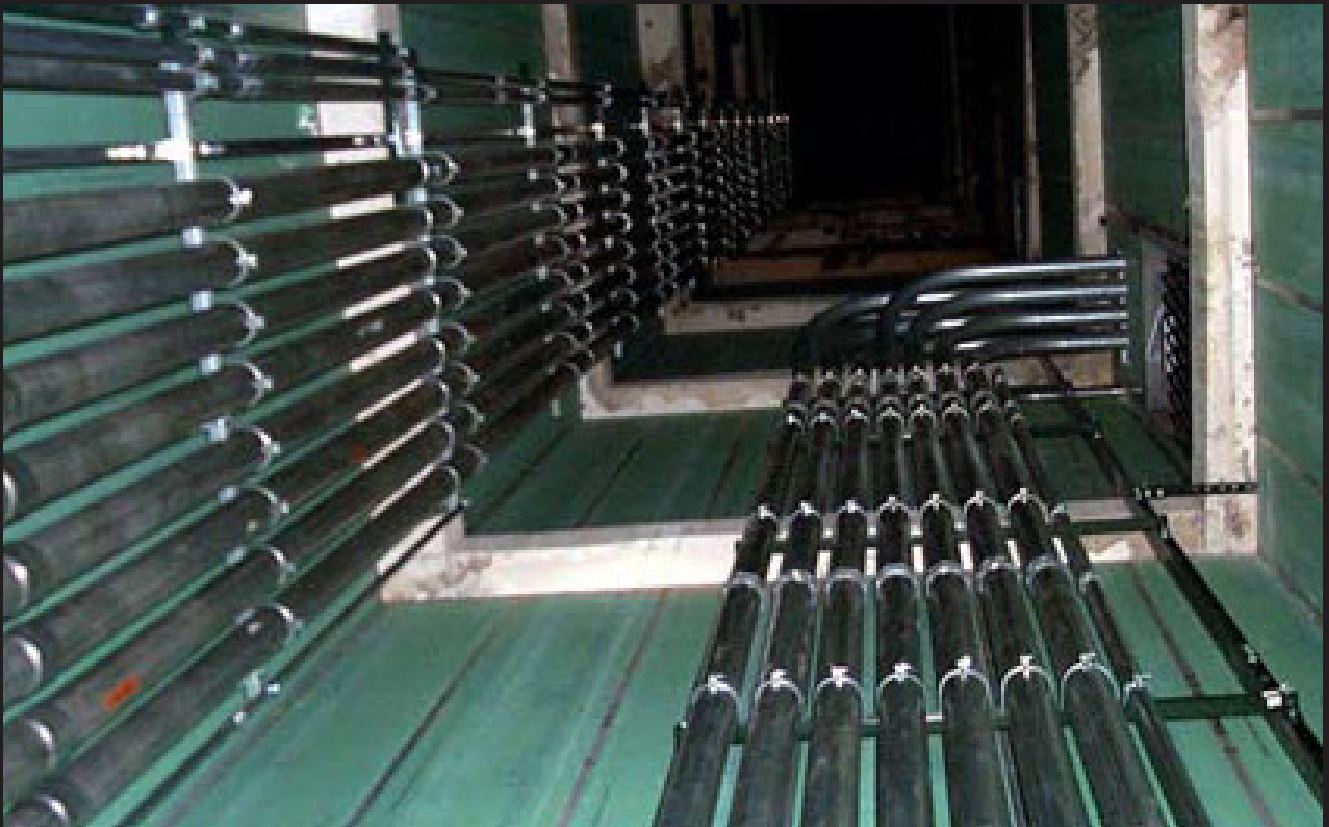
Fiber optic Risers - 350 E Cermak [Image 09]
