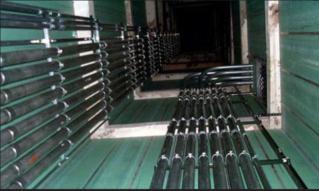
350 E. Cermak Fiber Optic Risers [Image 06]
