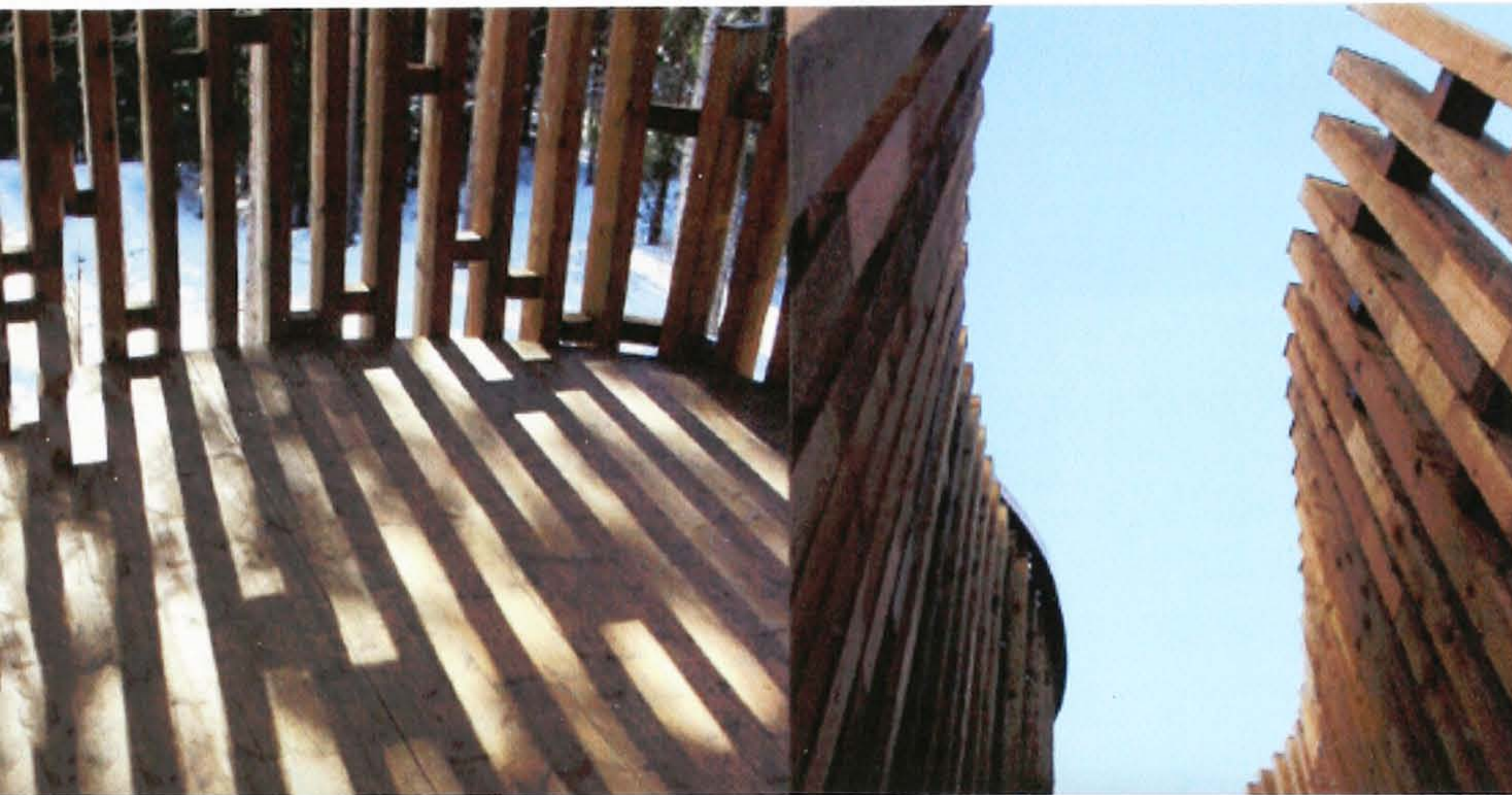
VIEWING TOWER SOURU, FINLANDE
