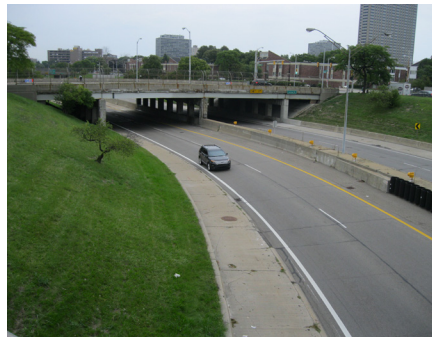
(fig.04) I-375 North-East View from Jefferson Ave.
