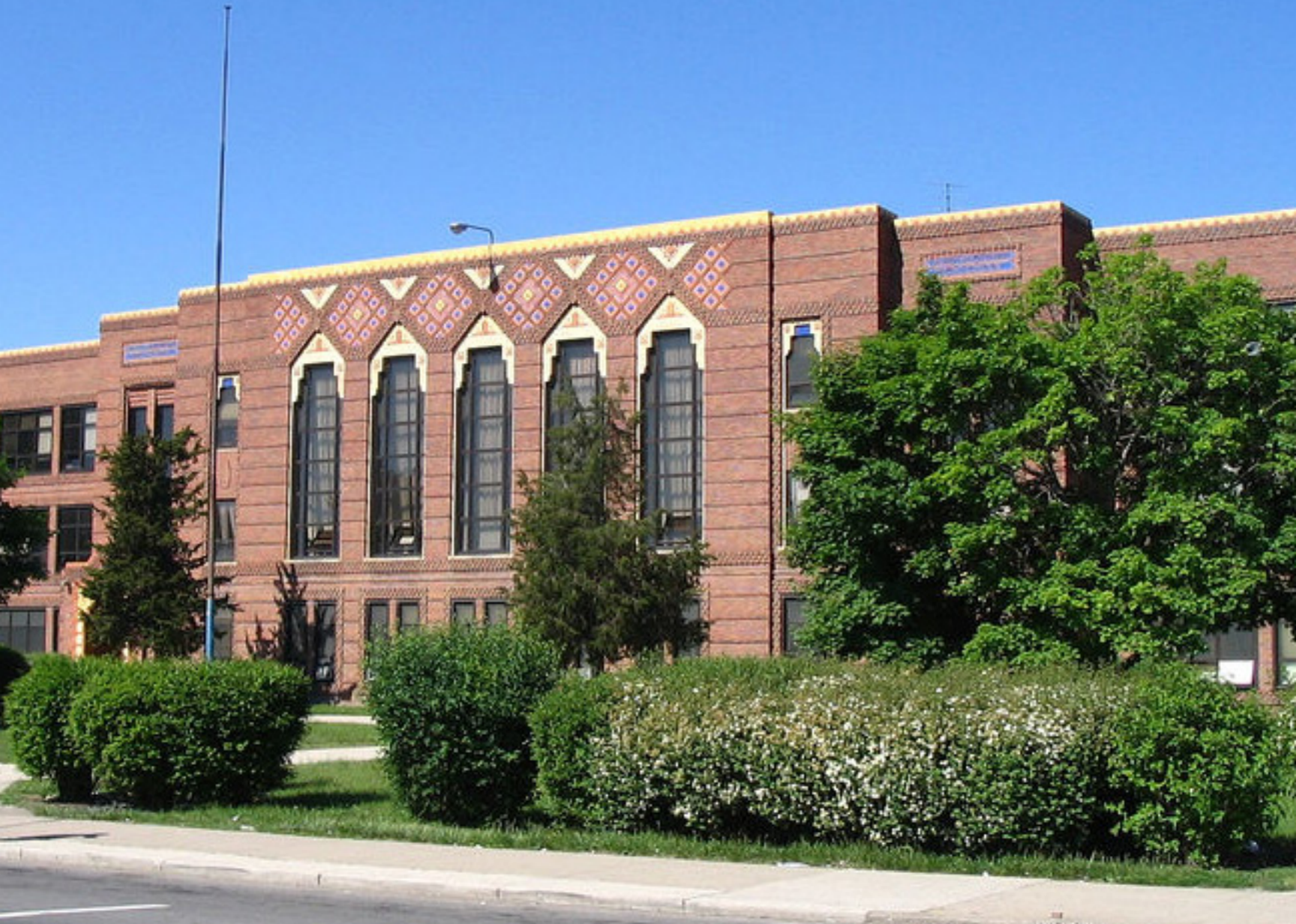
Mackenzie High School in Detroit, Michigan, built 1927. Designed by Wirt Rowland. Demolished 2012 (Makeloveland.com)
